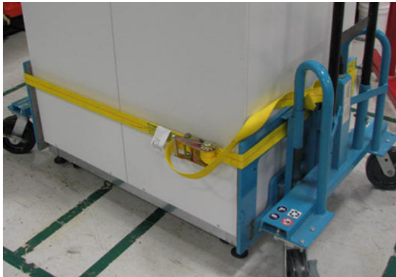
Figure 2-13 Securing the cabinet on the dolly
