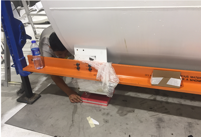
Figure 7-9 Lowering the magnet onto the vibroacoustic damping mats
