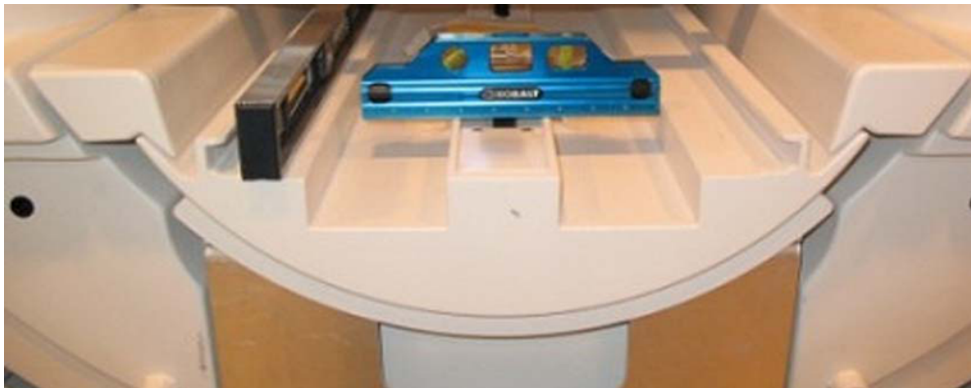
Figure 7-15 Magnet leveling, left-to-right
