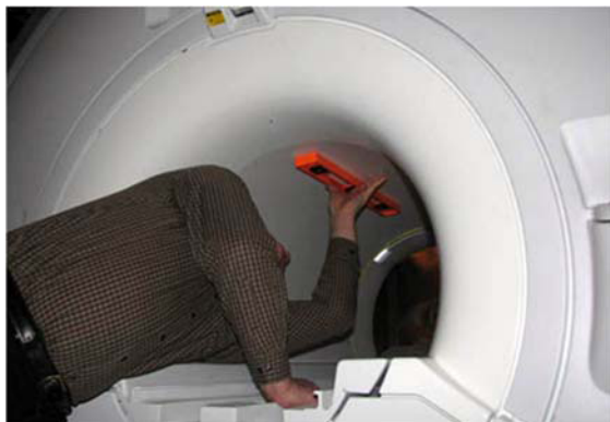
Figure 6-12 Magnet leveling, front-to-back
