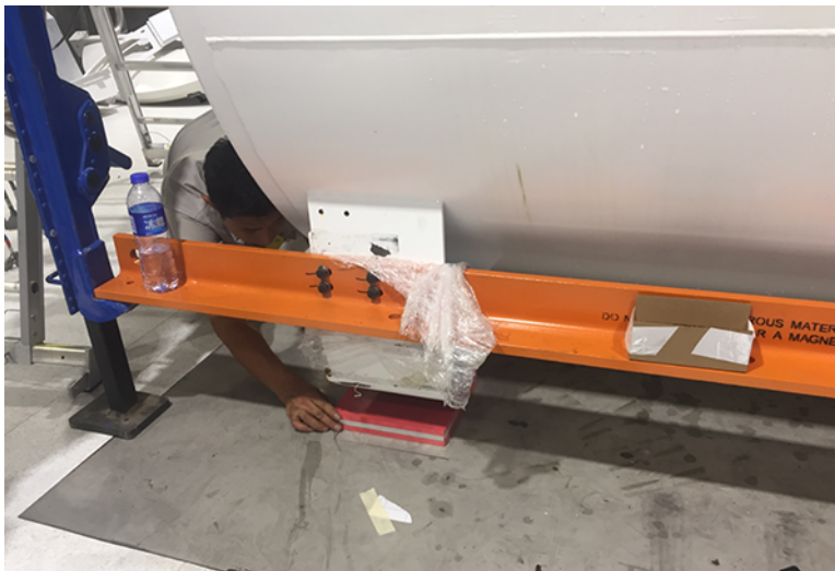
Figure 6-10 Lowering the magnet onto the vibroacoustic damping mats
