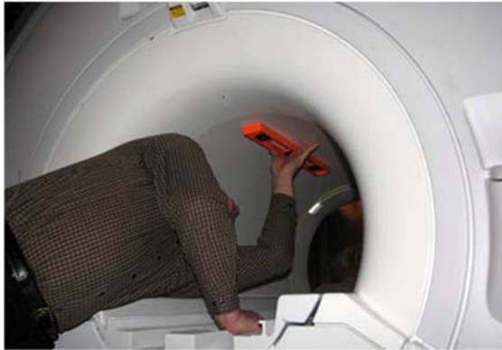
Figure 7-12 Magnet leveling, front-to-back
