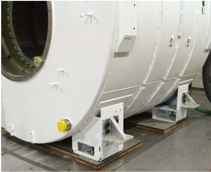
Figure 7-9 Magnet installed on surface mounted vibroacoustic damping mats*
