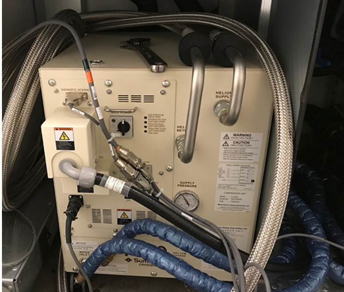
Figure 3-22 Arranging the hose insulation
